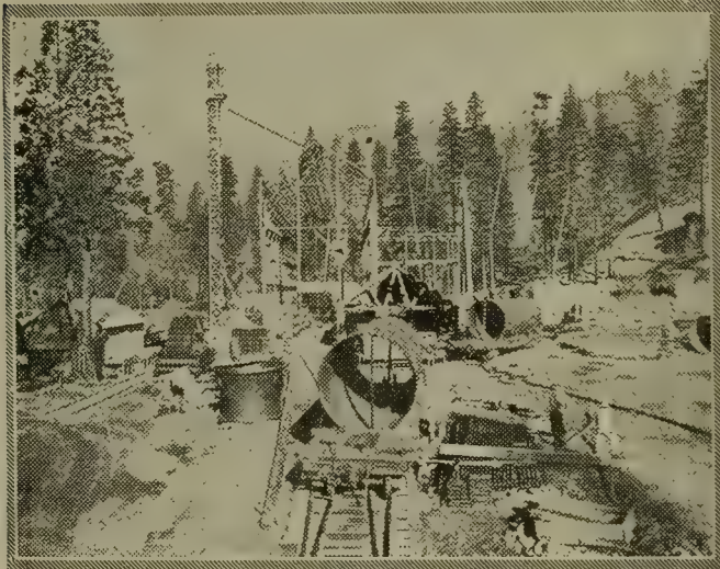
RAPID PROGRESS ON BIG POWER HOUSE
